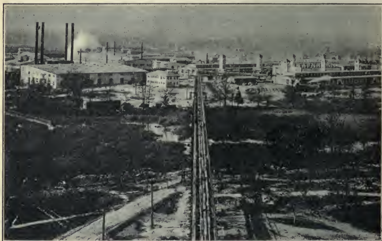
FIG. 19.—Chlorine Plant, Edgewood Arsenal.
